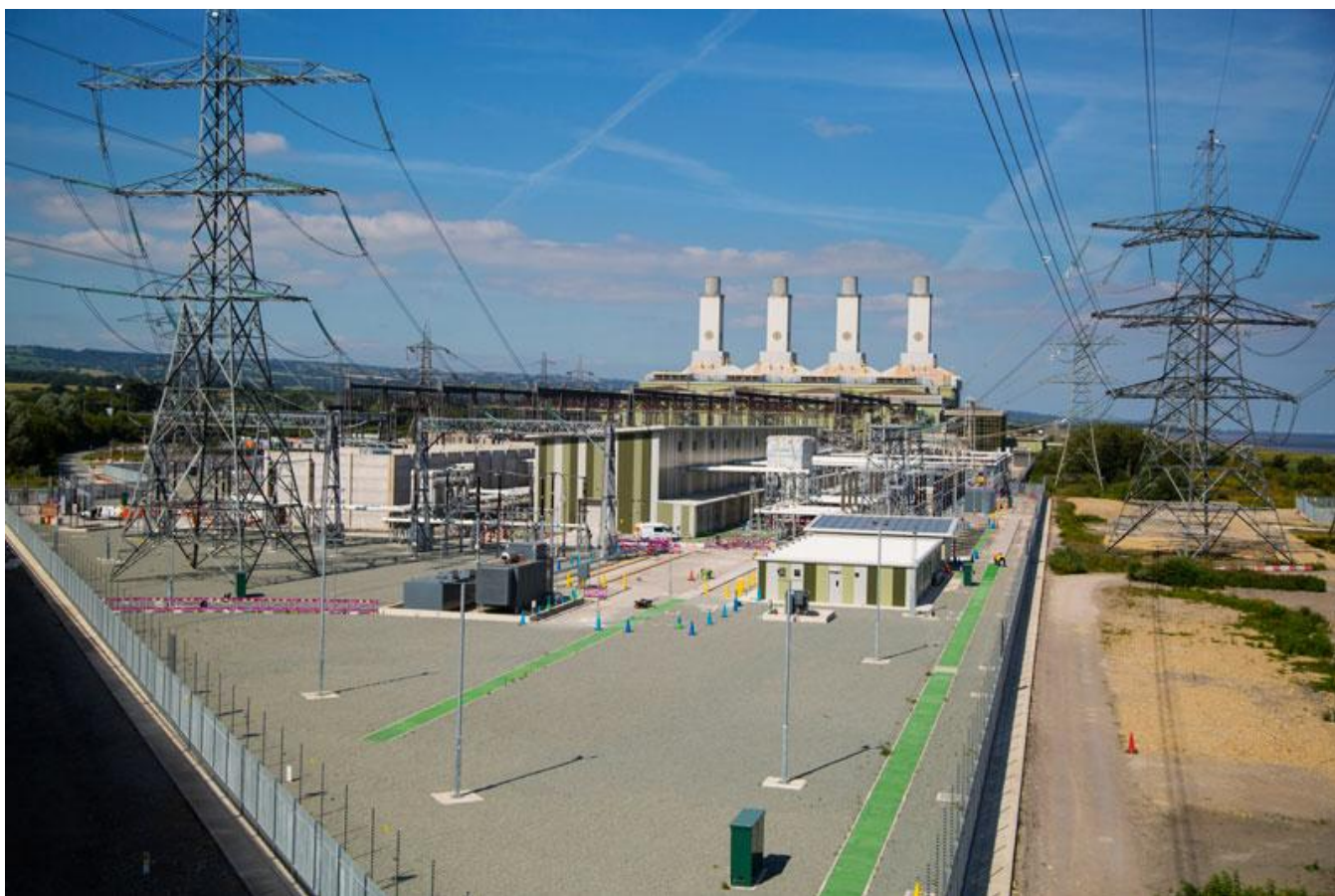
Image 3.4 Existing Connah's Quay 400 kV Substation in colour cladding (Source: National Grid)
