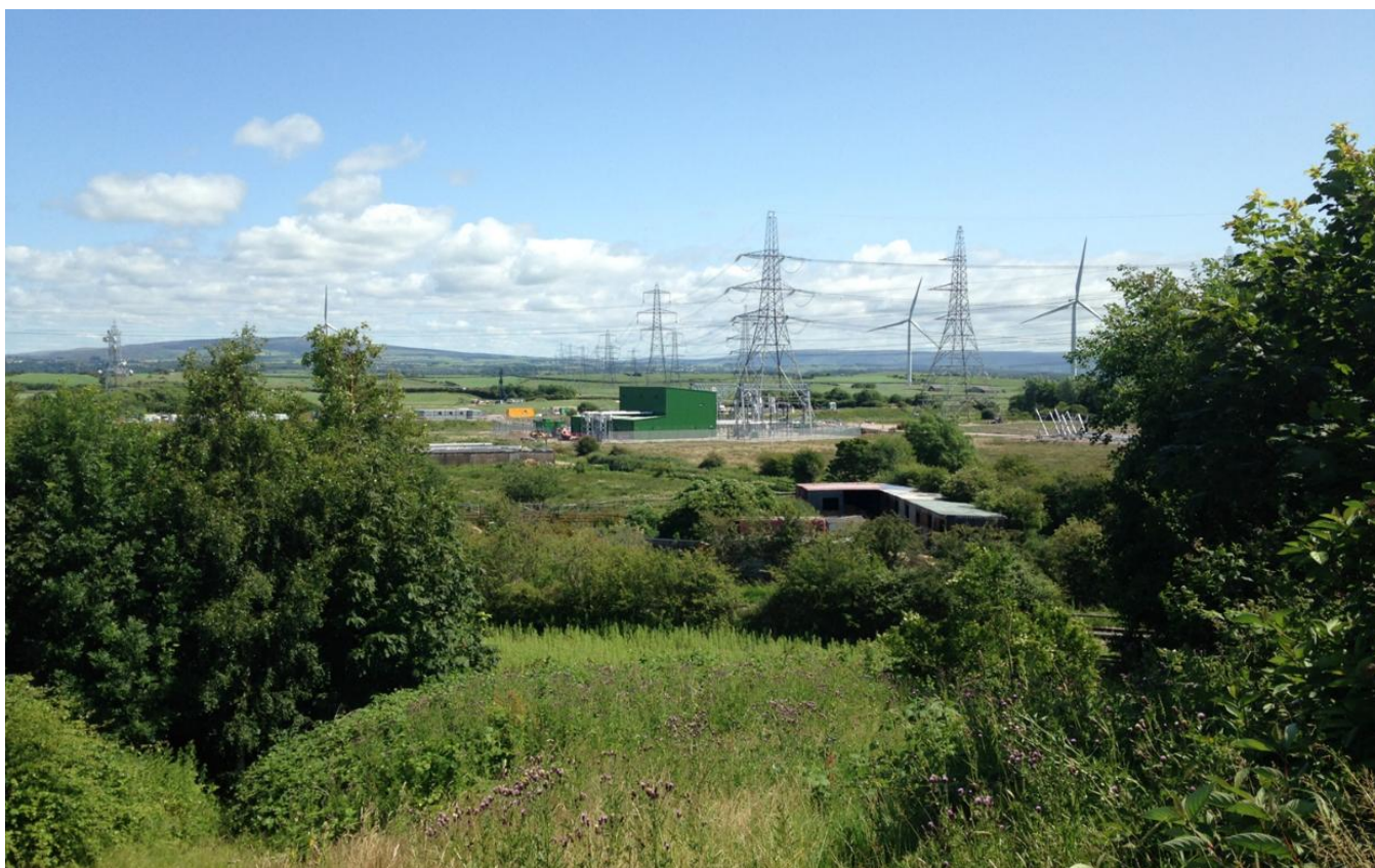
Image 3.5 Existing Middleton 400 kV Substation (Source: National Grid)
